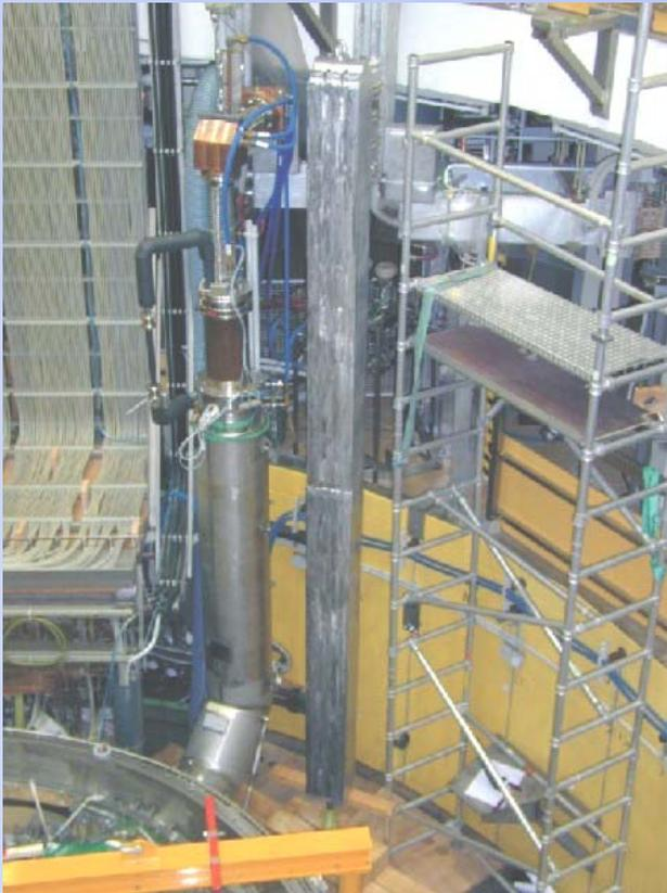
**Conventional 80 kA CL and Aluminium bus bar installed in TOSKA**
